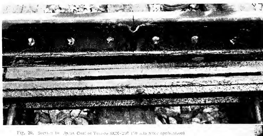
Fig. 20. Section 10, Spray Coat of Texaco RCX-208 (50 min after application)
